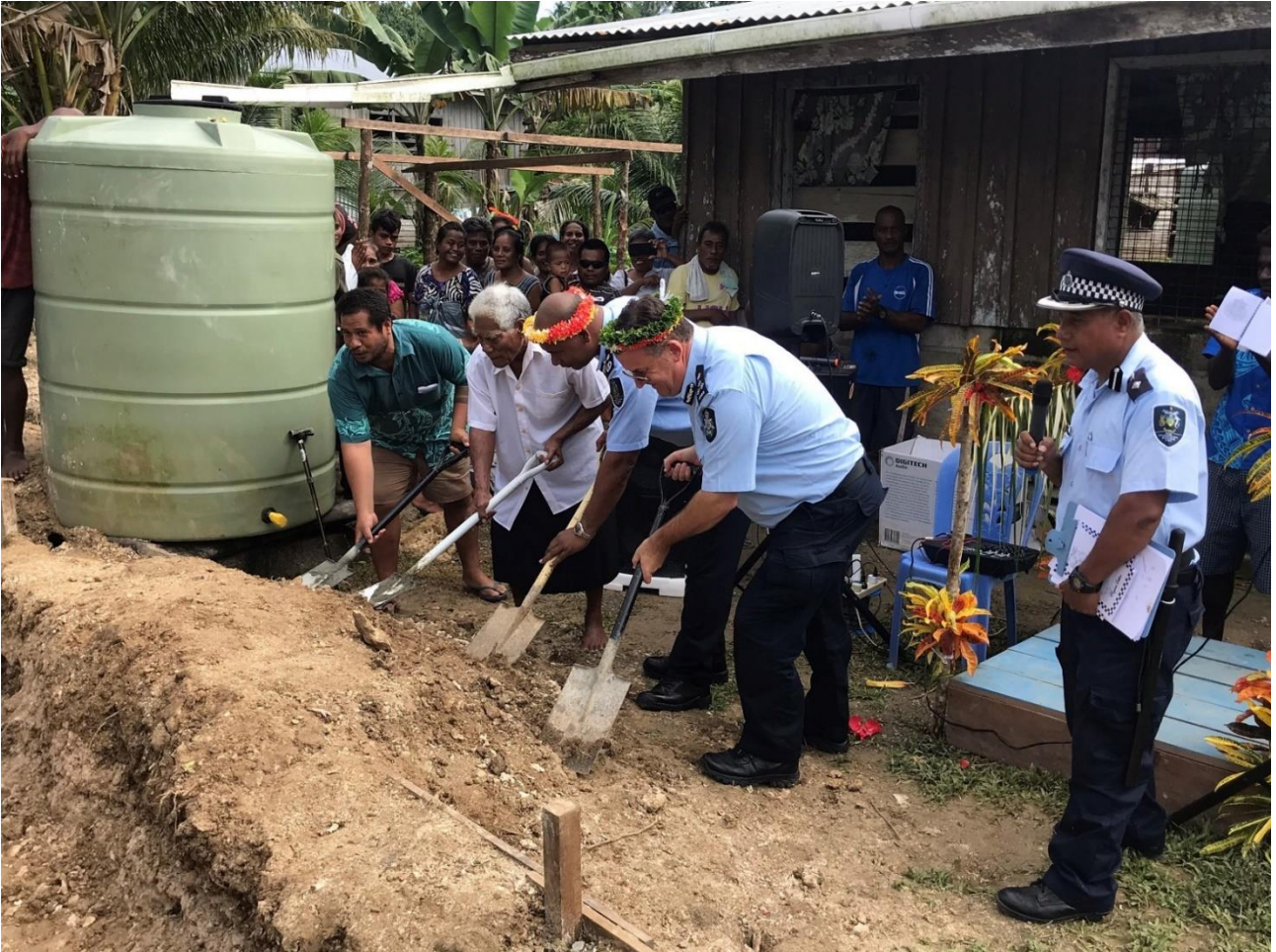
Turning of the soil at one of the sites
